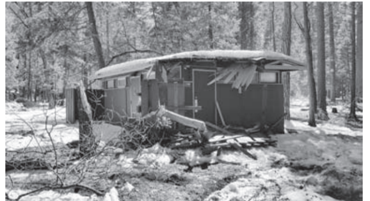
In this photo released Wednesday, March 13, 2019, by the National Park Service, is a damaged building after the recent heavy snowpack in Yosemite National Park, Calif.
